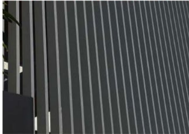
VERTICAL LOUVRES (LVR) POWDER COAT ALUMINIUM (INTERPON D2525 SABLE BRILLIANCE MATT) - TO MATCH CL1
